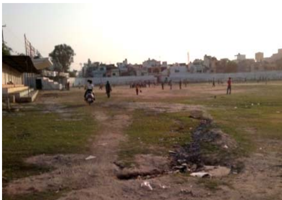
Fig. 8: Poorly maintained ground, Nehru stadium, Roorkee
