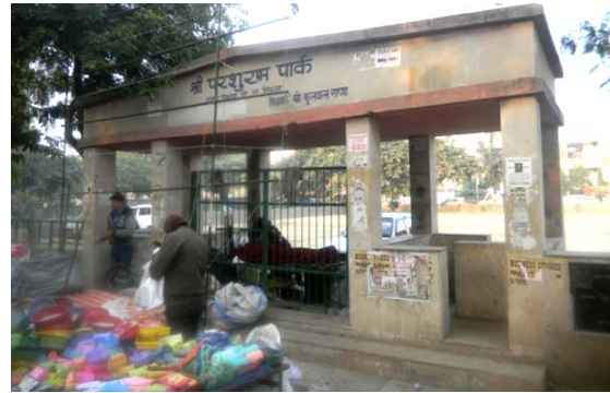
Fig. 14: Poor design and badly maintained entrance to park, Delhi
